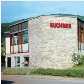
Production location in Unterböhringen
