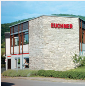
Production location in Unterböhringen
