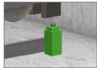
Switch for slack rope monitoring (governor rope)
